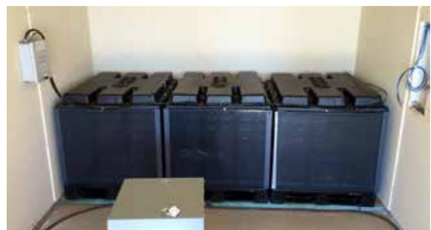
Figure 9: Three AHI M100 Battery Modules (60 kWh)
